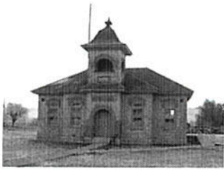
Fairfield School House, 1898
