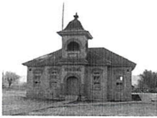
Fairfield School House, 1898
